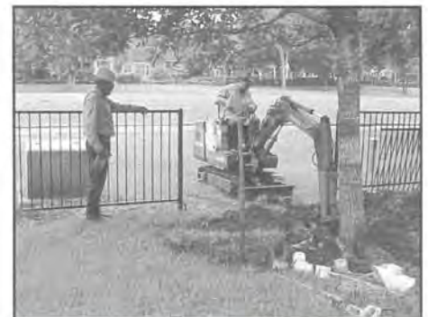
Paul Segura, Field Crew Leader (on tractor), and Jose Nunez checking sewer tap on the main line in easement.
