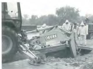
Water crew working on main line repair.
